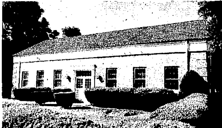
SLATED FOR EXPANSION... The Scotch Plains United States Post Office will be expanded to include a post office box section along with a "postal store" for retail postal products. Construction, which is set to begin this Saturday, July 5, will continue through the remainder of the year.
