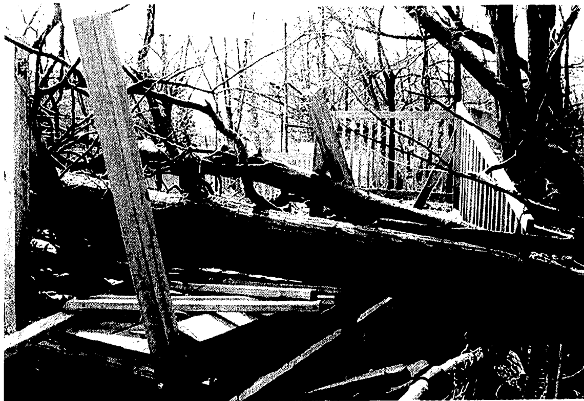
CRUSHED! ...Last week's heavy winds caused this large tree to fall on the dugout on the Scotch Plains-Fanwood Youth Baseball Little League Association's field. Although the dugout itself is made of concrete, the wooden viewing area directly behind it sustained substantial damage. This area is utilized by those persons who wish to take photographs or videotape games.
