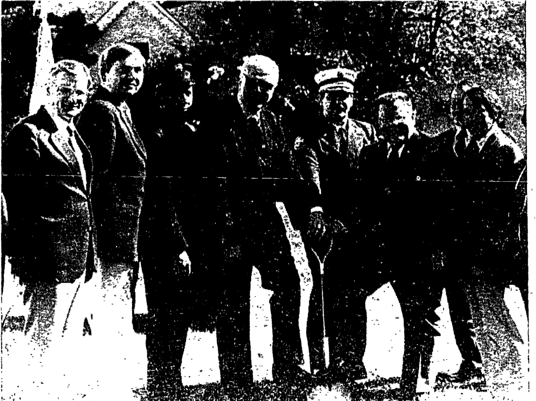
Turning the first shovel of earth for the new Fanwood firehouse are, left to right, Councilmen Andy MacDonald and Dave Charzewski, Fire Company President Robert Scala, Mayor Ted Trumpp, Fire Captain Russ Hamill, Councilmen Doug Clausen, Paul Abbott and Robert Rau, Jr.
