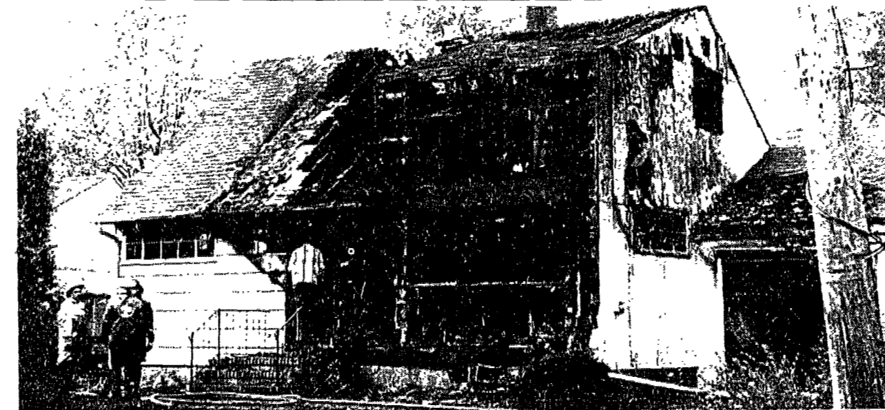
Fire gutted house where mother and two young children died.
