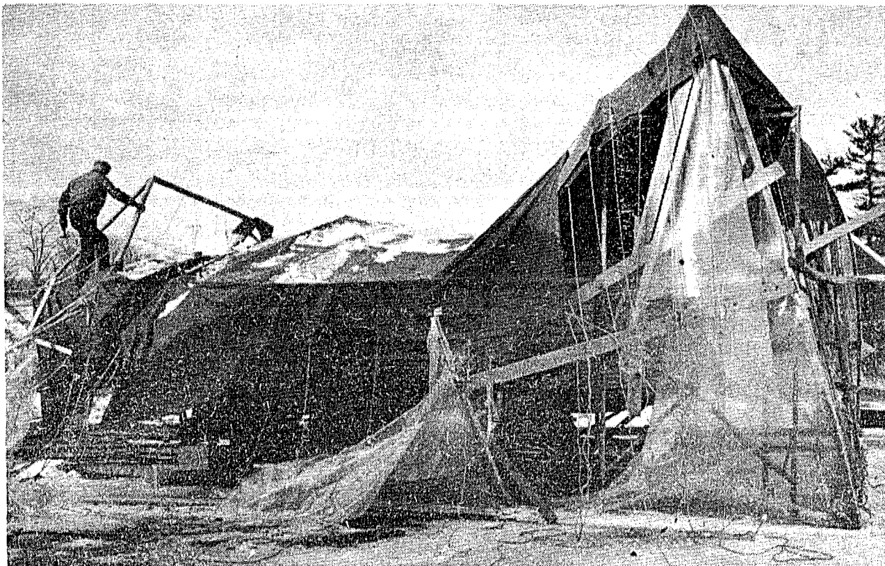
Last weeks wind and snow storm all but demolished the protective structure built by the Sea Scouts to shelter their 34 foot boat.
