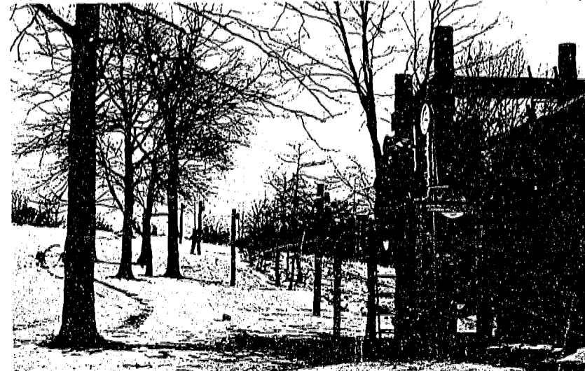
SKI TOW READY TO GO—650 foot ski tow at the Galloping Hill Golf Course receiving finishing touches from Union County Park Commission maintenance crews. The tow will be in operation with first good snowfall.
